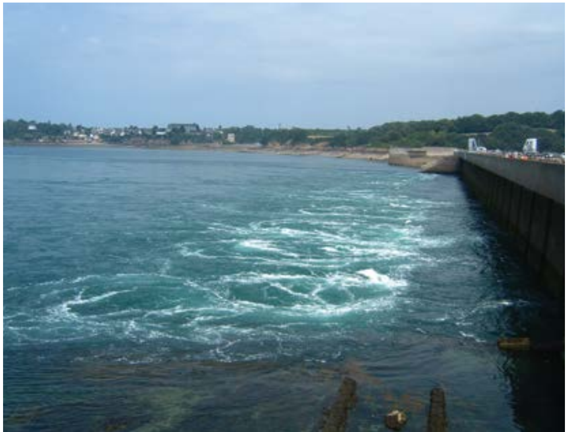
FIGURE 10-21 (Right) La Rance tidal power-generating plant in France.
