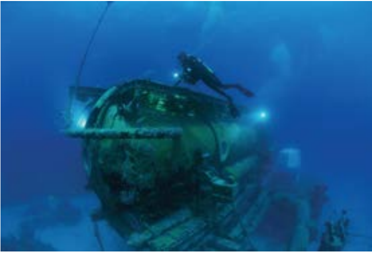
FIGURE 3-20 Underwater habitats, such as Aquarius, shown here in the Florida Keys, enable scientists to live and work up to several tens of meters underwater for several days without incurring decompression sickness. However, at the end of their stay they must undergo very long decompression periods in a decompression chamber.
