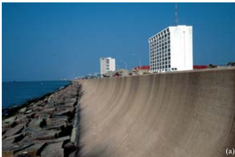
FIGURE 11-21 Seawalls are designed to protect beachfront property from erosion. (a) The Galveston seawall was constructed after the destructive hurricane of 1900. Since the wall was completed in 1962, the beach has eroded along much of its length, leaving the shoreline more exposed to attack by the highest waves of future hurricanes. (b) The barrier island has continued to retreat since the Galveston seawall was constructed. The beach just beyond the end of the wall has now retreated substantially farther shoreward than the wall's location as a result of the natural process of barrier island retreat and the consequent reduction in the amount of sand in the littoral drift system that occurred once the beach had been eroded away in front of the wall. (c) Seawalls are undermined from the sides and eventually destroyed as sea level rises
